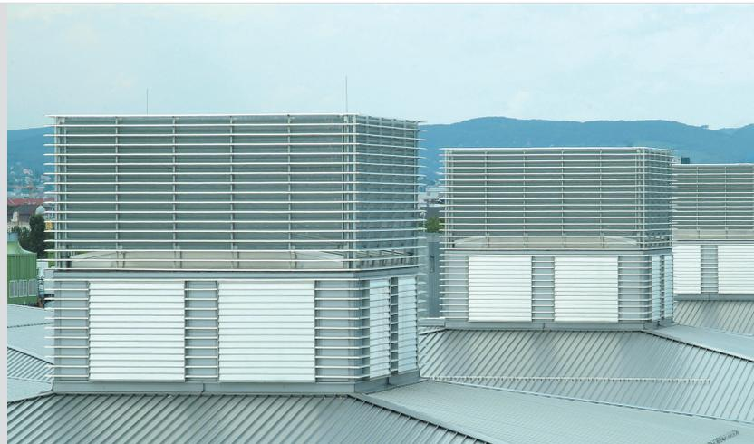
action locking mechanisms, failsafe open or failsafe closed. If used as either an electric or a pneumatic smoke ventilator, activation is either by local thermal fuse which opens the unit at a pre-selected temperature, or by responding to an external release signal.
